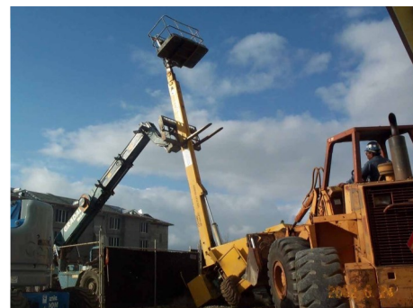
Gradall & loader support aerial lift
